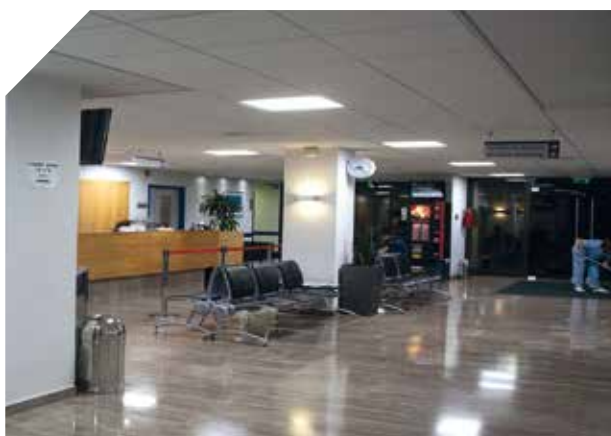
Reception lights application.
